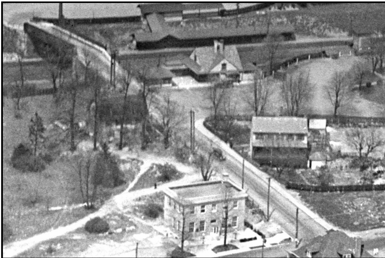
In this photo taken in 1926, the Wedge Building, shown in the foreground, sits on the northwest corner of Lancaster Pike and Valley Road, just south of the Paoli PRR station. Behind it is a three-story building with Dutch-style roof, which at one time was used by the Pennsylvania Railroad to change-over its steam engine crews. In the 1920s it was owned by the Great Valley Mill. Directly across Valley Road was one of the oldest landmarks in Paoli, the Canal Collector's Office of the Main Line of Public Works, which dated to the late 1830s. Courtesy of Hagley Museum and Library, and Tredyffrin Easttown Historical Society.
