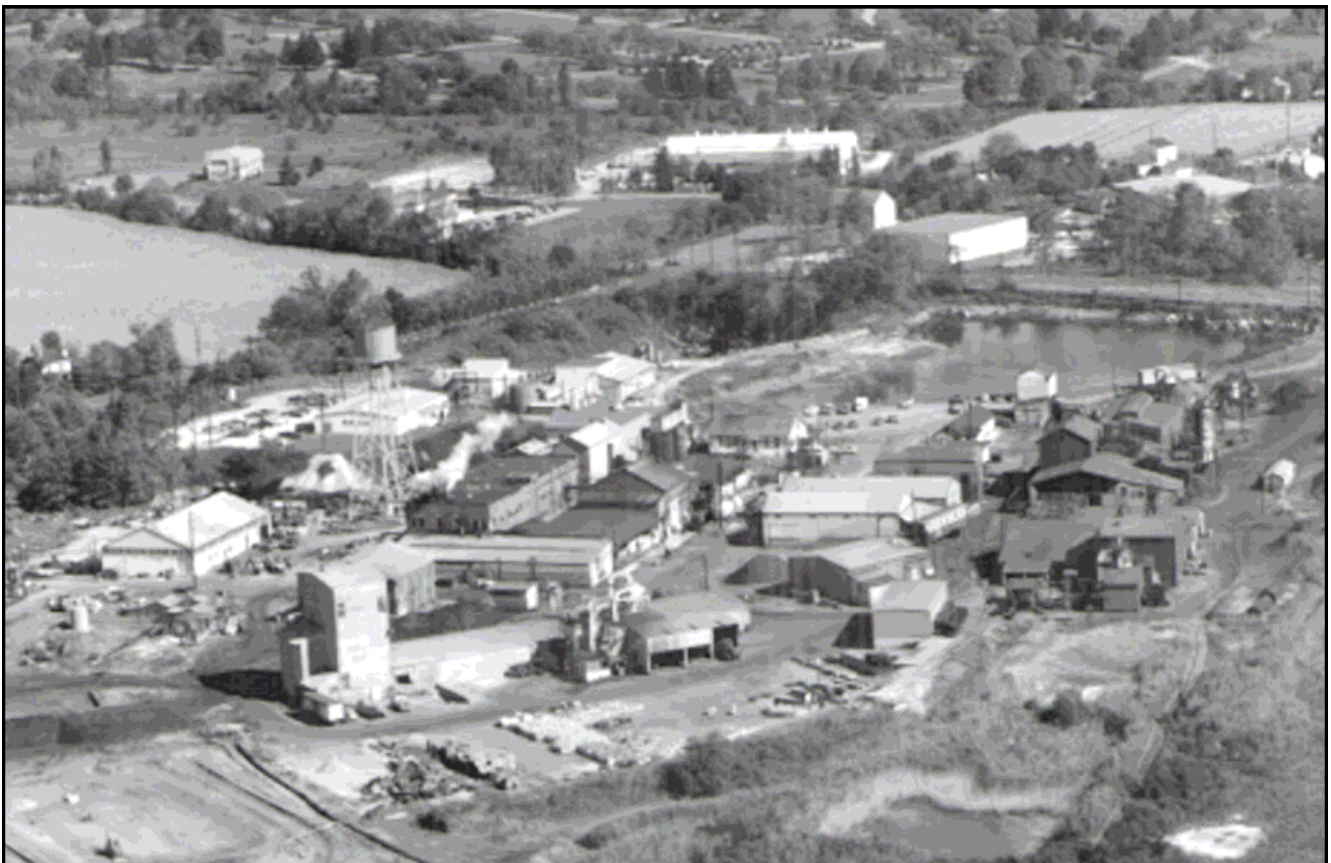
Looking north, an aerial view of the Foote quarry site in East Whiteland Township in the 1940s. Photo courtesy of the author.
