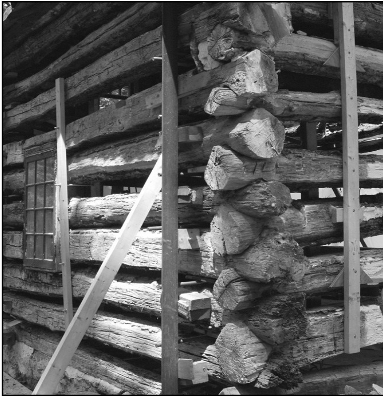
The unique characteristics of inverted V-corner notching, and the “crowning” beyond the points of attachment, indicated original construction of the Church Road Cabin before 1790. Courtesy of Roger D. Thorne.
