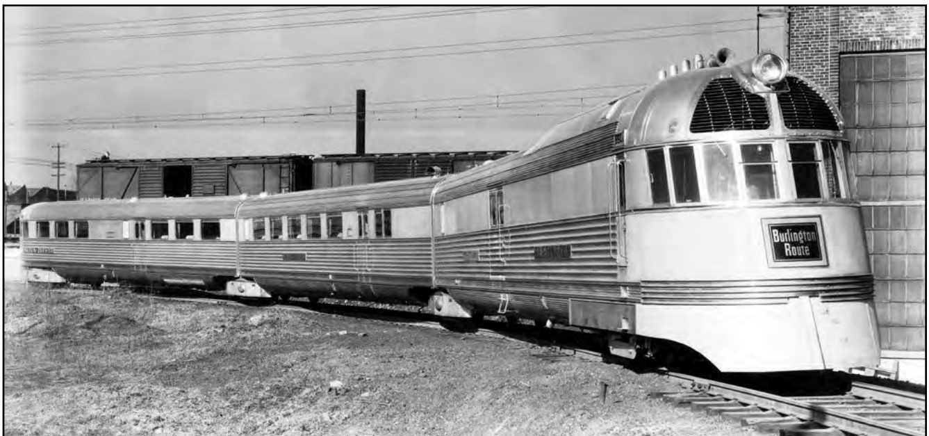
The stainless steel, streamlined Burlington Zephyr, completed by the Edward G. Budd Manufacturing Co. in Philadelphia for the Chicago, Burlington & Quincy Railroad, is powered by a Winton diesel engine, and is America's first diesel, all-steel streamlined train. Courtesy of Temple University Libraries, Urban Archives, Philadelphia, PA.
