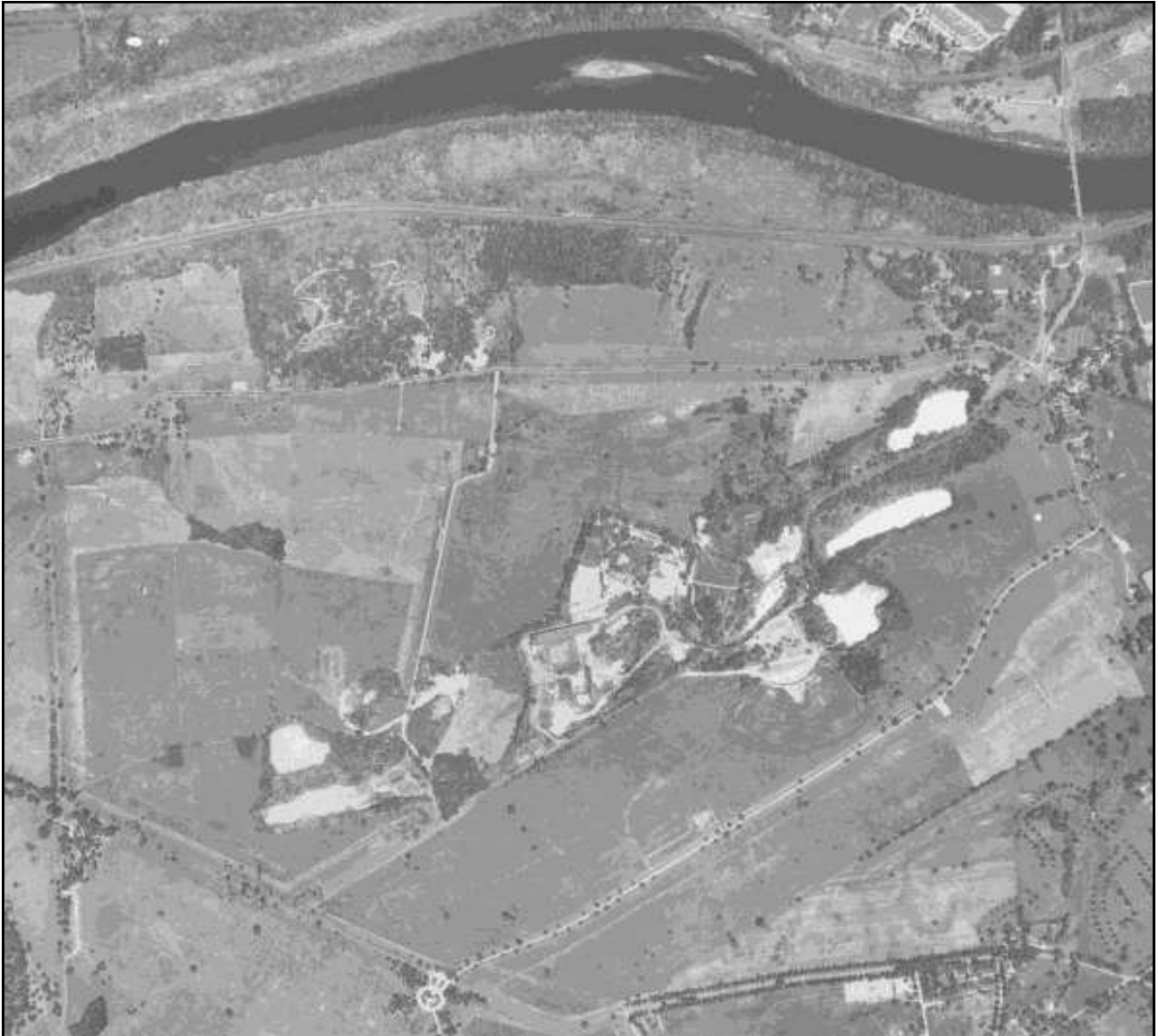
A 1958 aerial photograph showing quarries filled with asbestos waste (white areas). Photo from http://www.pennpilot.psu.edu
