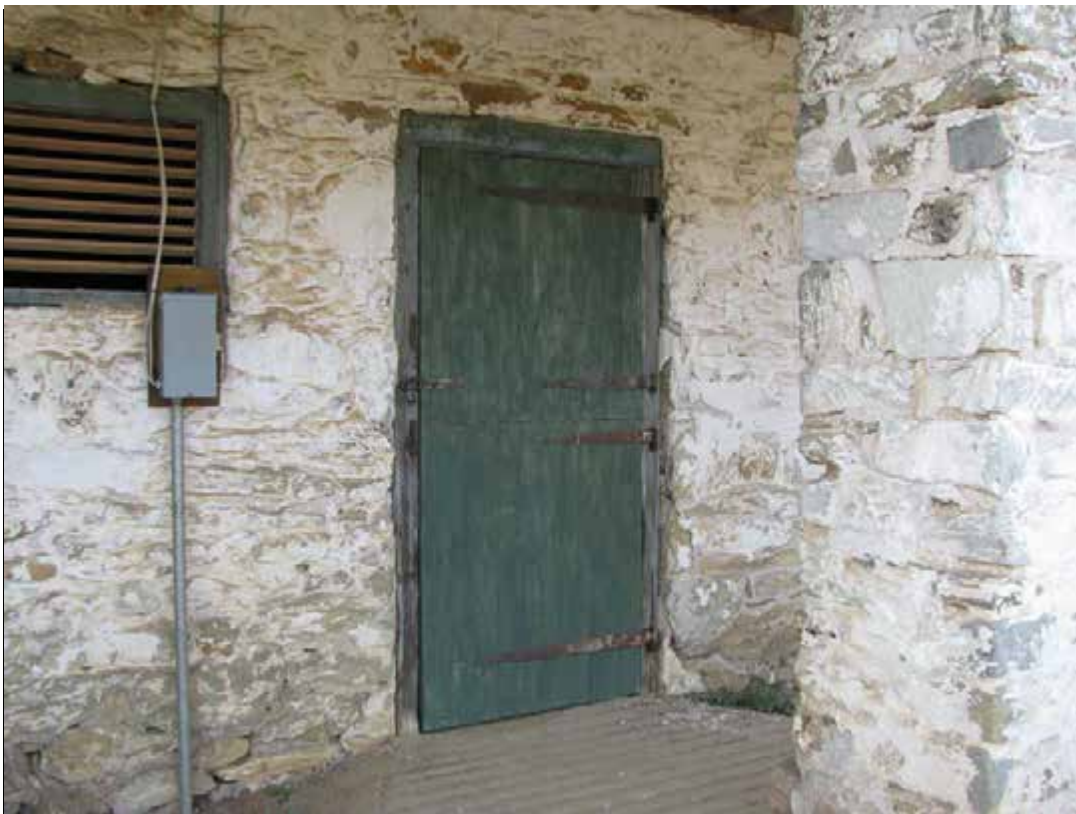
Above: This ground level “Dutch” door located in the forebay provides access to the stable area. The door, hinges, and nearby window are all new to the Federal Barn. One of the stables, although unrestored, remains in fairly good shape. Below: A window well on the north side of the barn, with the new concrete foundation just below it.
