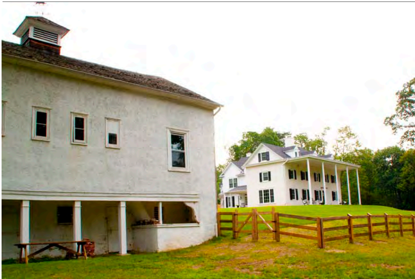
A contemporary view of the renovated Buttonwoods house and barn originally owned by the Patten family. Courtesy of Dave Reid.
