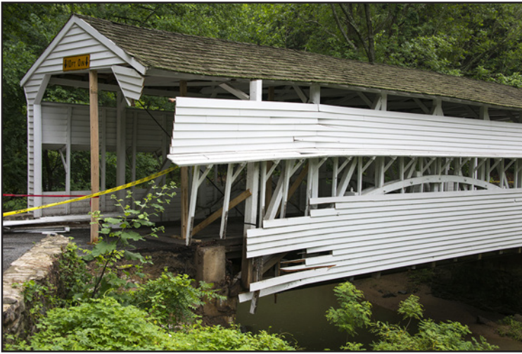
ABOVE: Collision damage to the Knox Covered Bridge, 7 July 2015.
