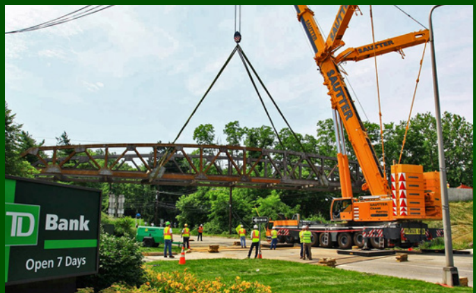
ABOVE LEFT: 24 June 2013 – The assembled bridge framework, hooked-up and ready for lifting into place. The Liebherr LTM1400-7.1 crane provided by Sautter Crane Rental, capable of lifting 485 tons, is the second-largest in the eastern U.S. ABOVE RIGHT: 25 June 2013 – The lifting process: slowly and very carefully moving the 60-ton structure into position.
