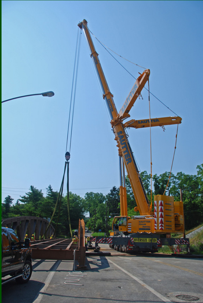
ABOVE LEFT: 24 June 2013 – The assembled bridge framework, hooked-up and ready for lifting into place. The Liebherr LTM1400-7.1 crane provided by Sautter Crane Rental, capable of lifting 485 tons, is the second-largest in the eastern U.S. ABOVE RIGHT: 25 June 2013 – The lifting process: slowly and very carefully moving the 60-ton structure into position.
