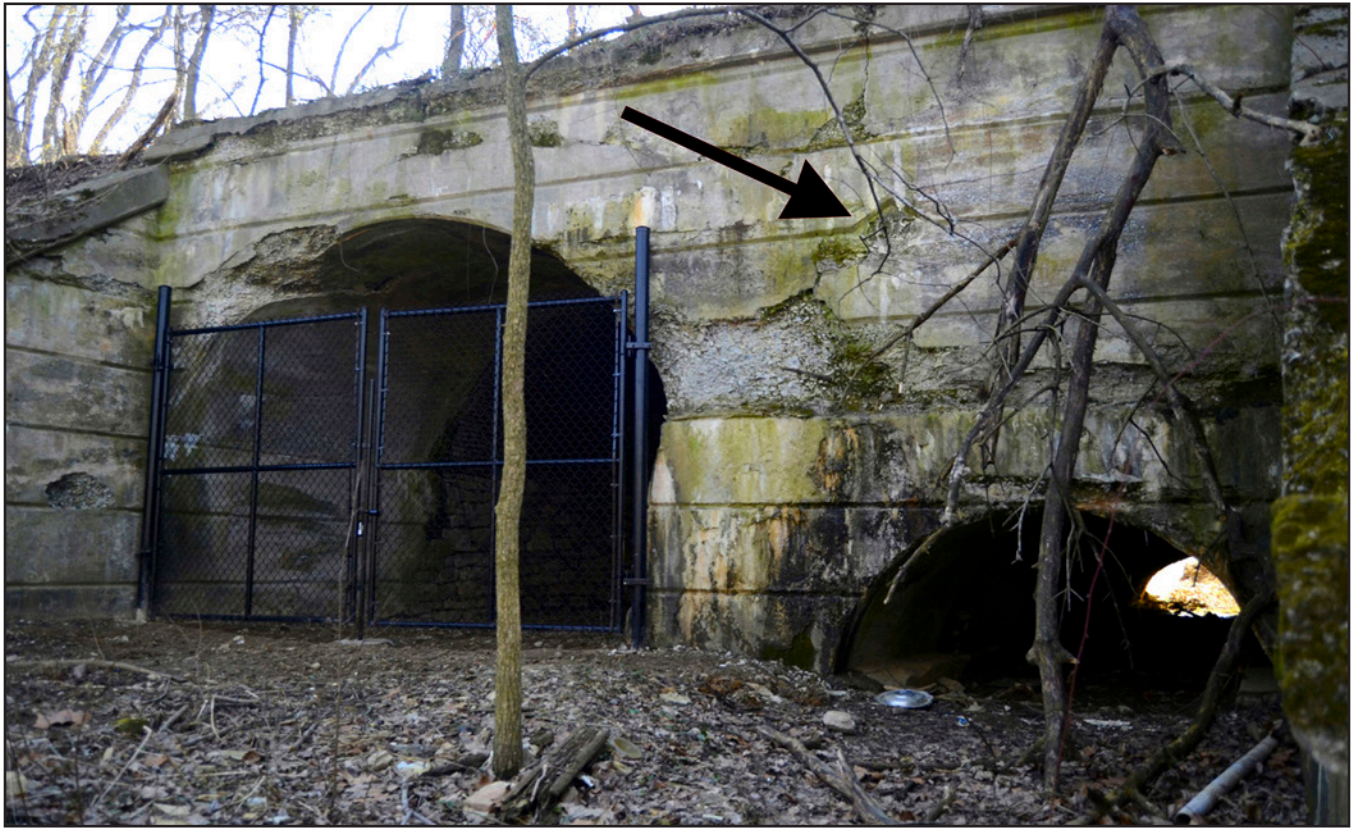
North face of ChVRR Farm Road Underpass No. 14 at Howellville. The larger portal on the left was for wagon traffic, and the smaller culvert at right for a mill race off Crabby Creek. Arrow points to the obscure P&R “1917” Diamond in the concrete facing located between the portals. Photographed in 2011 by Roger D. Thorne.
