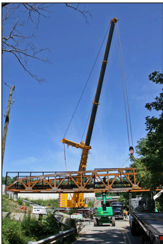
A Pratt truss bridge being lowered into place over North Valley Road. Work was performed over a weekend in August 2013. Photo by Tim Lander.
