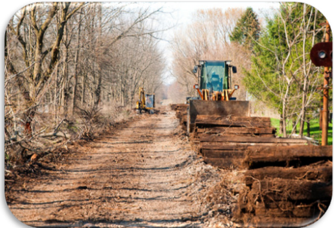
Rails and ties are removed as part of the abandonment process. Photo courtesy of Chester County Department of Facilities and Parks.
