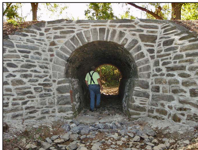
A member of the county bridge maintenance staff inspects newly repaired Culvert #11, west of West Valley Road. Photo courtesy of Chester County Department of Facilities and Parks.
