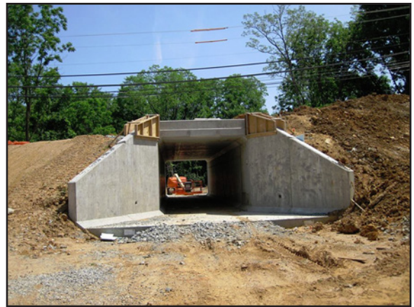
Box culvert under Warner Road. Photo by Tim Lander.
