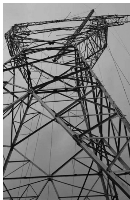
An electrical transmission line tower under construction, with a gin pole visible near the top.
