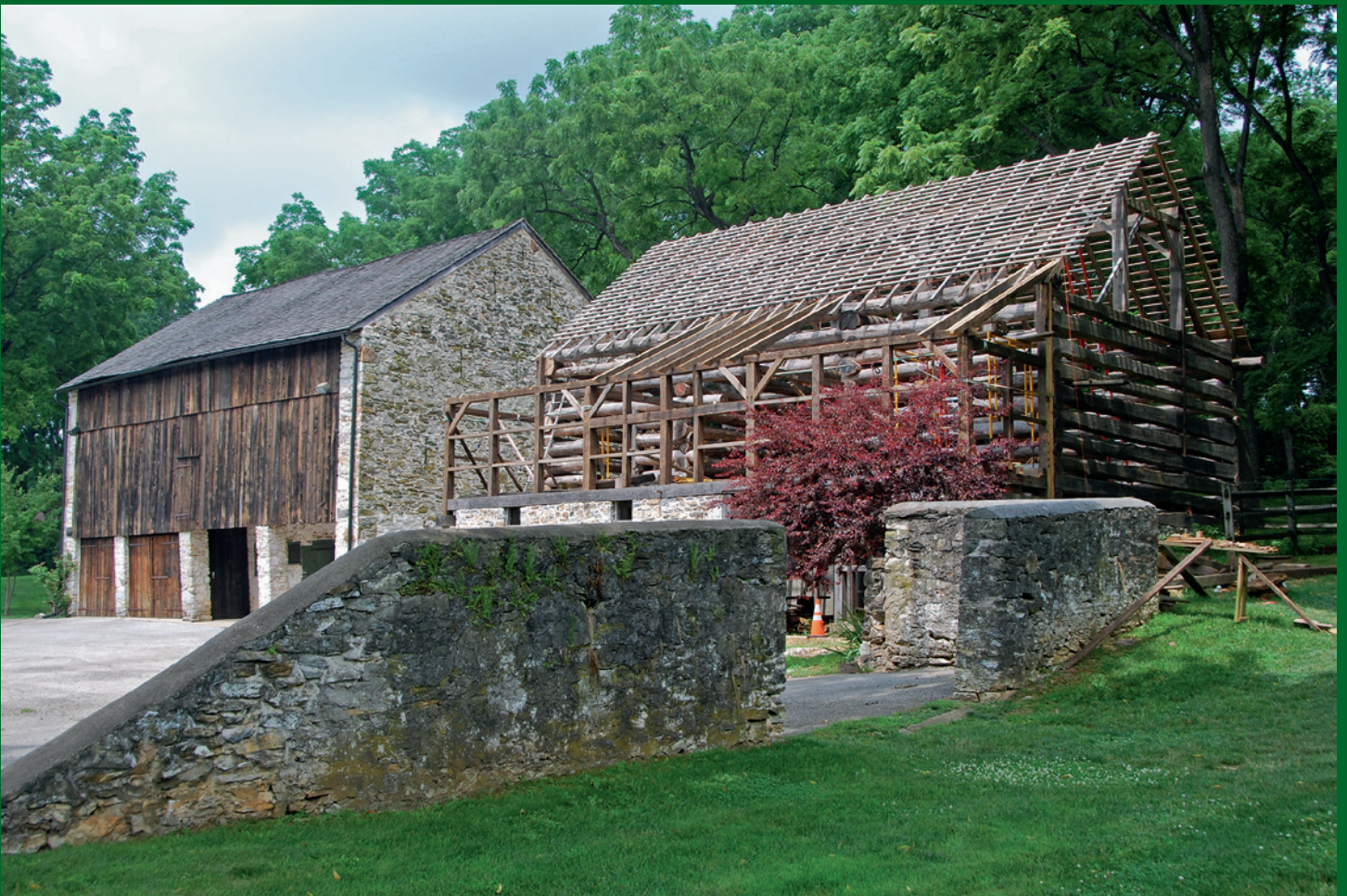
The framing of the roof and front section takes shape in the spring (May 2019).
