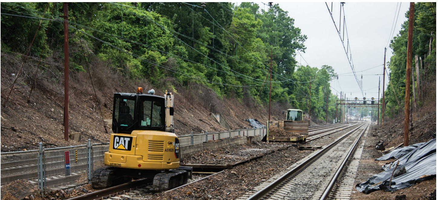
Track work east of Paoli station, photographed on May 30, 2017, in preparation for the construction of the Paoli Transportation Center. This image reminds the reader of the reality of the "cut" initially constructed for two tracks in 1876-77, in places rising as high as 28 feet above the tracks, and finally widened to its current four-track size in 1893. This "cut" extends from Bear Hill Road (currently Route 252) west past North Valley Road. Courtesy of Roger D. Thorne.
